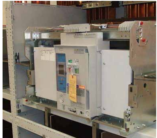
Figure 1.0: Modern Low voltage Air Circuit Breaker
